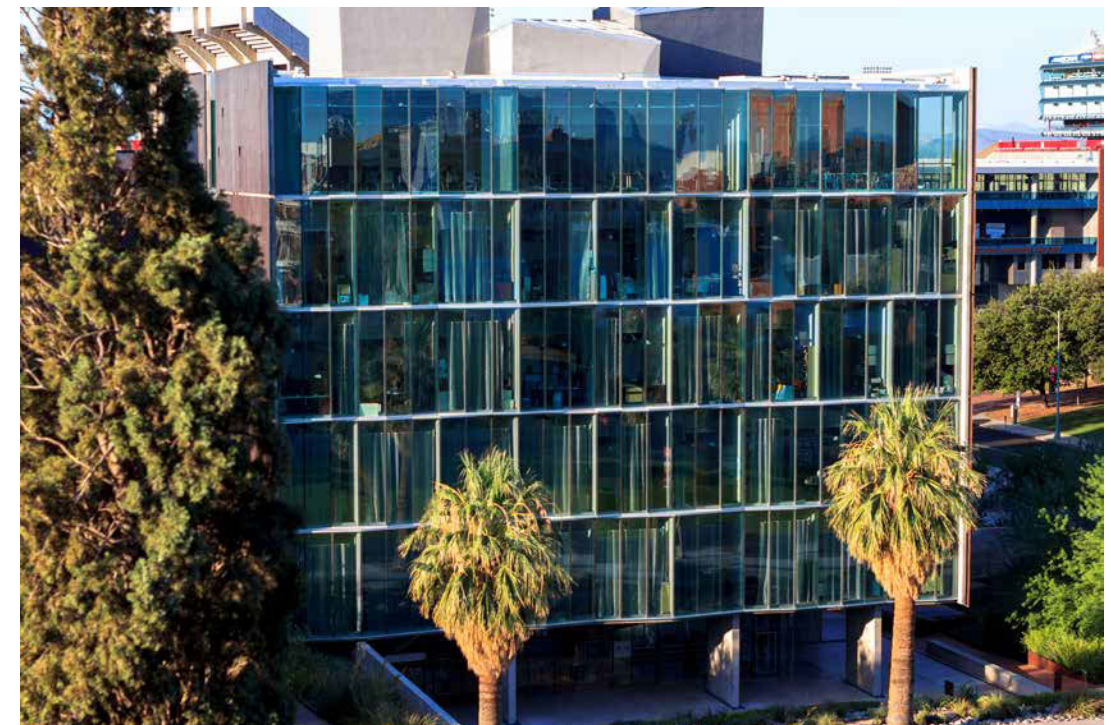
The north façade of the Meniel Optical Sciences Expansion
